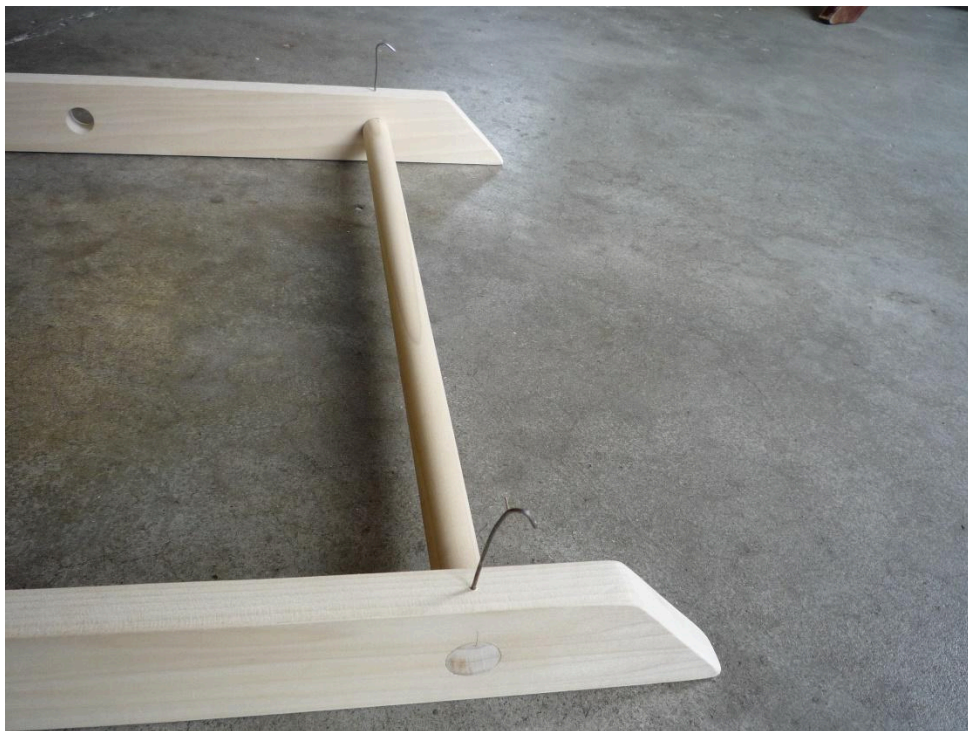
Temporarily pin the dowels to assist in positioning
